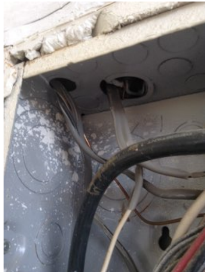
Cable clamps (sometimes referred to as bushings or grommets) are required where wiring passes into the main distribution panel. Cable clamps serve to protect the wiring from the metal edges of the panel openings.
