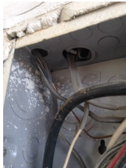
Cable clamps (sometimes referred to as bushings or grommets) are required where wiring passes into the main distribution panel. Cable clamps serve to protect the wiring from the metal edges of the panel openings.
