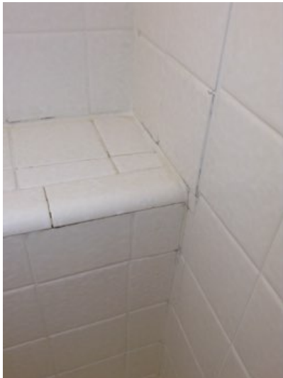
The tile shower stall requires repair. Loose or damaged tile, grout and caulk should be repaired or replaced as necessary. Any damage to the wall behind the tile should also be repaired (if necessary). Further investigation may reveal the need to rebuild a portion of the shower stall.
