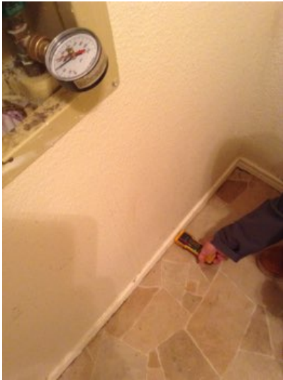
The laundry room wall and baseboard need to be repaired due to moisture damage.
