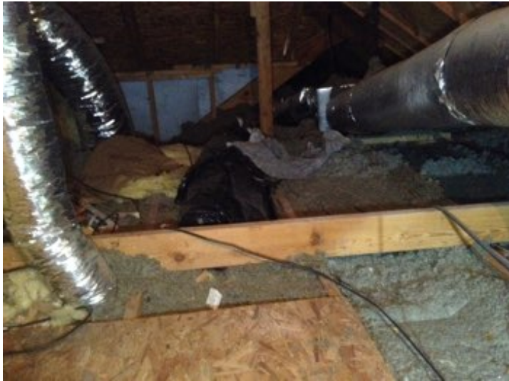
Insulation improvements are needed. The suggested depth of insulation on an attic floor is 10 to 12 inches of loose fill or an R-Factor of R-38 or more.
